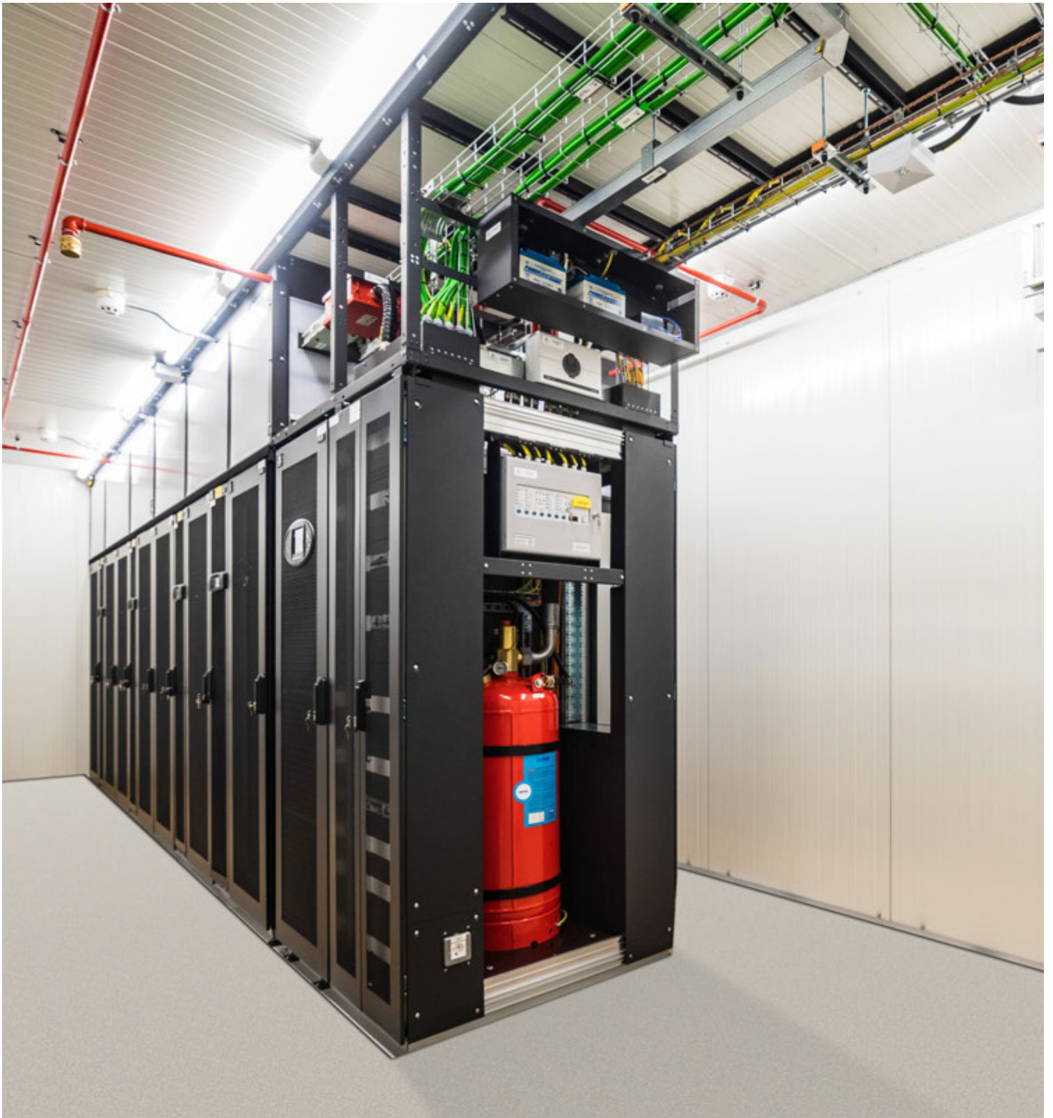
Interior view of SmartMod
